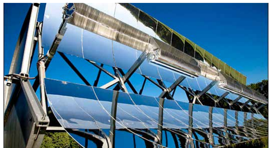
At KaXu Solar One, a solar power station in Pofadder, in the Northern Cape, the sun's energy is received by these parabolically curved trough-shaped reflectors.
