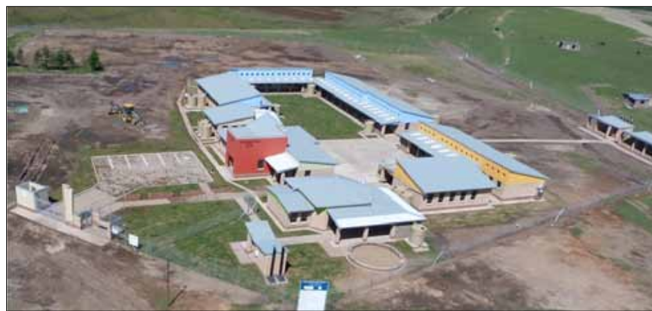
Tabata Senior Primary is one of the 10 new schools built in the Eastern Cape as part of the ASIDI.
