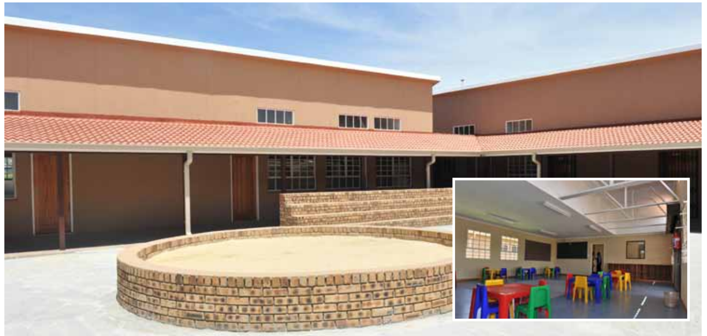
Newly-opened Orefile Primary in Olievenhoutbosch is the country's first environmentally friendly school and will offer a unique learning experience to its pupils. The Grade R classrooms (inset), which have toilets and sickrooms, are a burst of colour.
