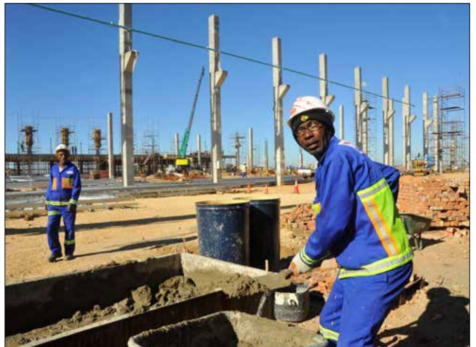
Sealing the deal: A worker on site at Chinese car and truck manufacturer First Automobile Works' (FAW) new plant in Zone 2 of the Coega Industrial Development Zone (IDZ).
