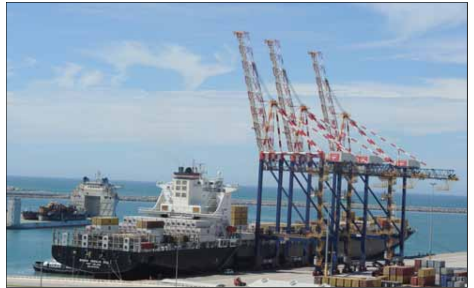
South Africa's ports are being upgraded as part of the country's massive infrastructure drive. The new Port of Ngqura in Port Elizabeth is the deepest container terminal in sub-Saharan Africa.
