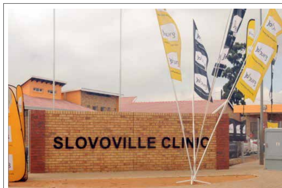
The newly built clinic in Slovoville means residents no longer have to travel to neighbouring communities to get quality health care.
