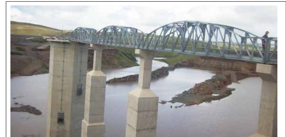
The newly constructed Ludeke Dam in the Eastern Cape is part of the Greater Mbizana Regional Bulk Water Supply Scheme, which will supply clean drinking water to about 270 000 people.
