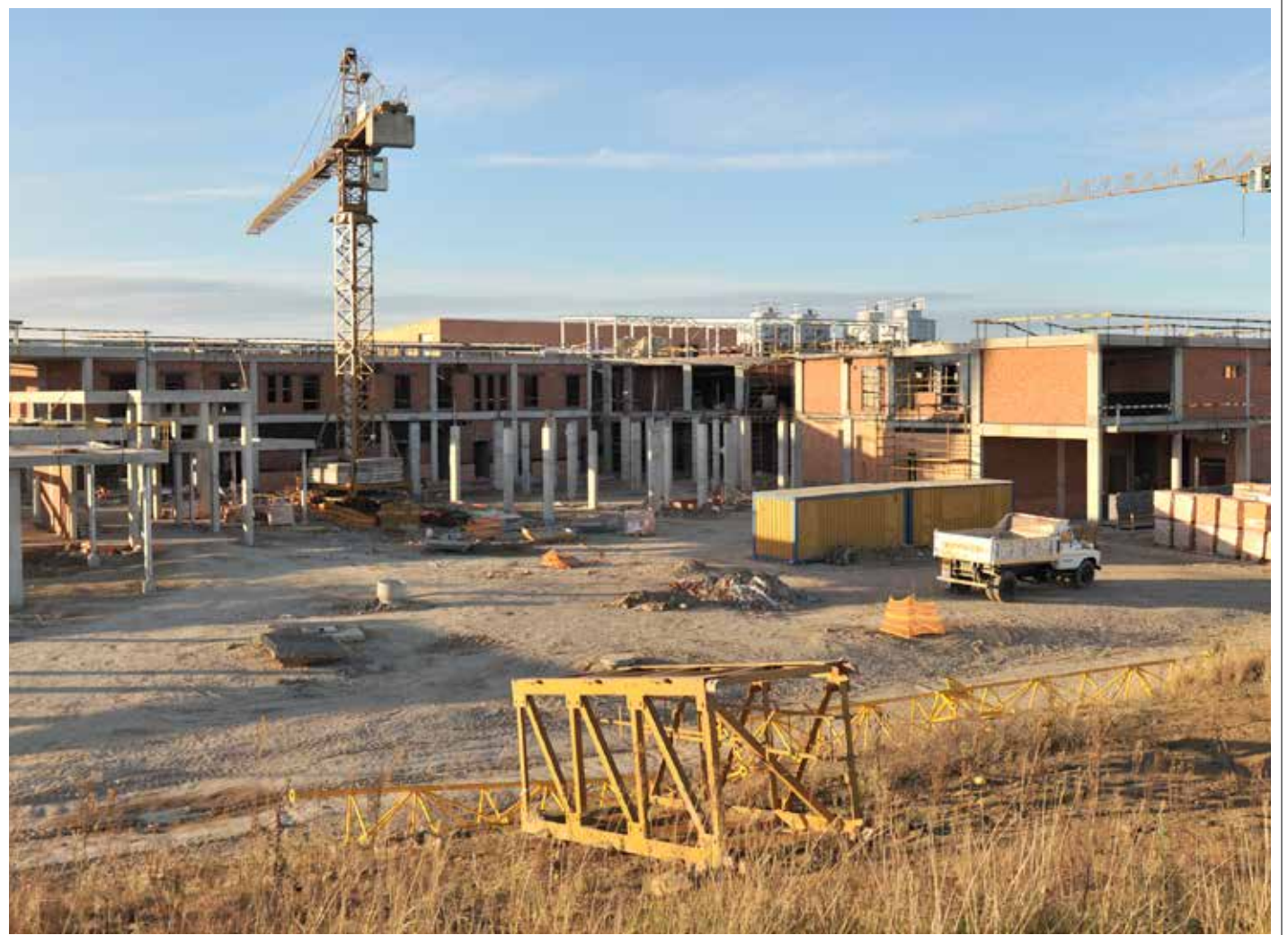
Construction of the new Cecilia Makiwane Hospital will be completed in 2017.
