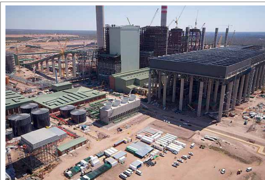
The Medupi Power Station is now expected to deliver power to the national grid in the middle of 2014
