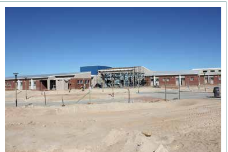
■ Construction on a new community health centre in Port Nolloth in the Northern Cape is almost complete. The facility will soon offer the small town greater access to healthcare services.
