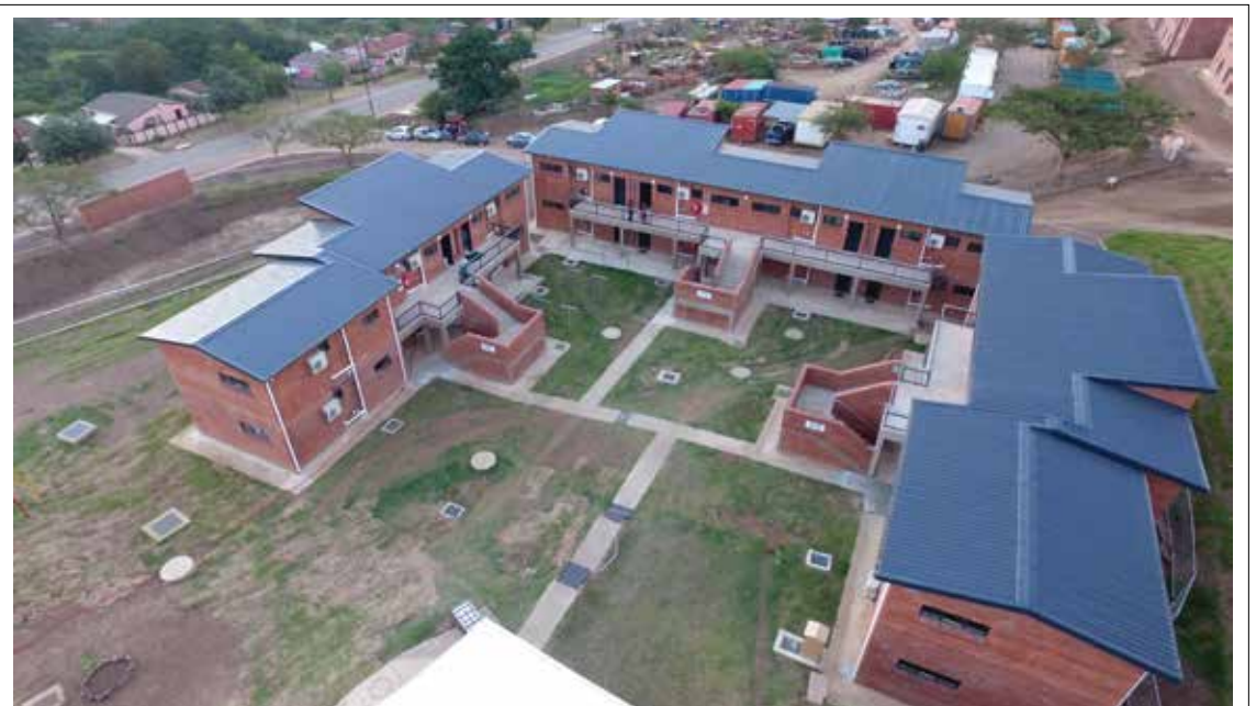
■ The Westgate housing project is expected to deliver close to 1 000 housing units, accommodating close to 4 000 beneficiaries once completed.
