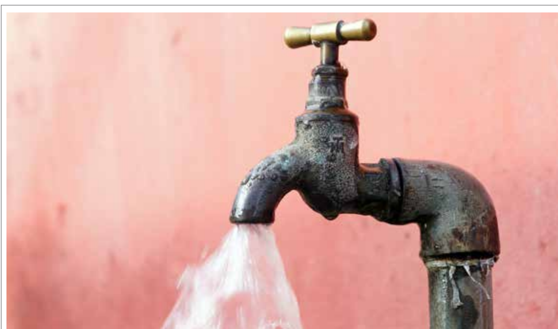
■ Leaking taps or potholes are some of the things that can be reported on the citizen Engagement App.
