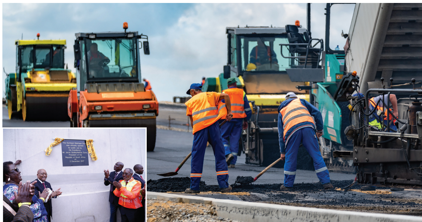
■ Dumisani Makhaye Drive is the biggest road infrastructure development in the country in five years.
