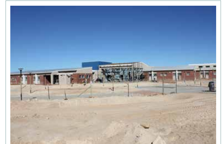
■ Construction on a new community health centre in Port Nolloth in the Northern Cape is almost complete. The facility will soon offer the small town greater access to healthcare services.
