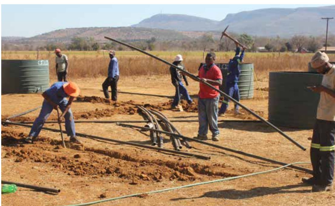
■ Fish Tank Reticulation System under construction in Hekpoort.
