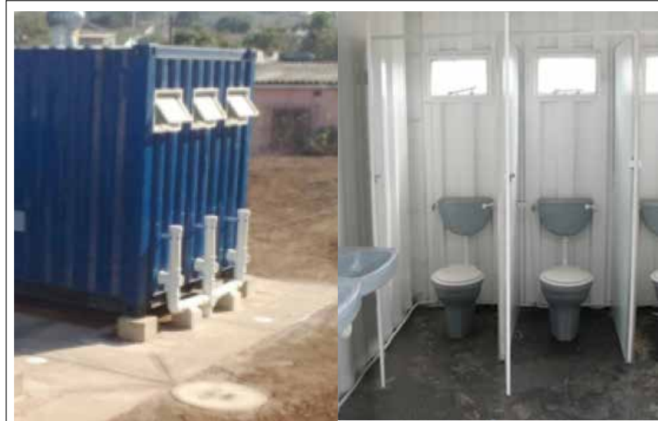
The eThekweni Municipality's Water and Sanitation unit uses modified ship containers to deal with the sanitation challenges in informal settlements in the province.
