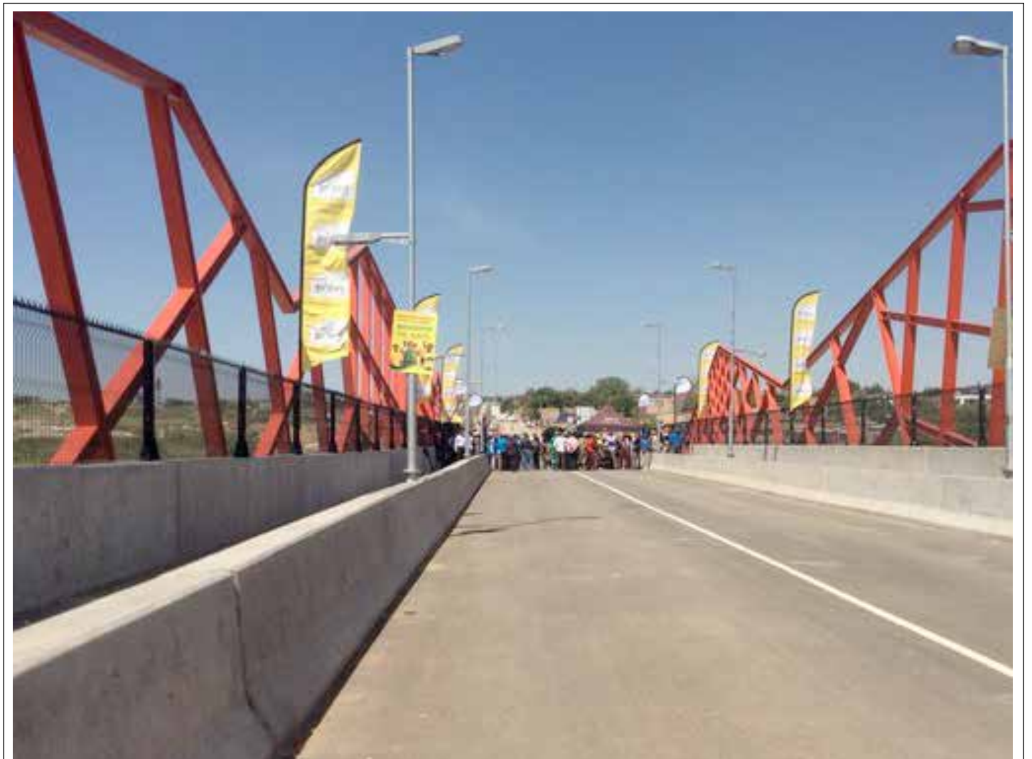
Diepsloot residents are benefiting from the new Ingonyama Bridge that helps them to commute between their home and work places safely.
