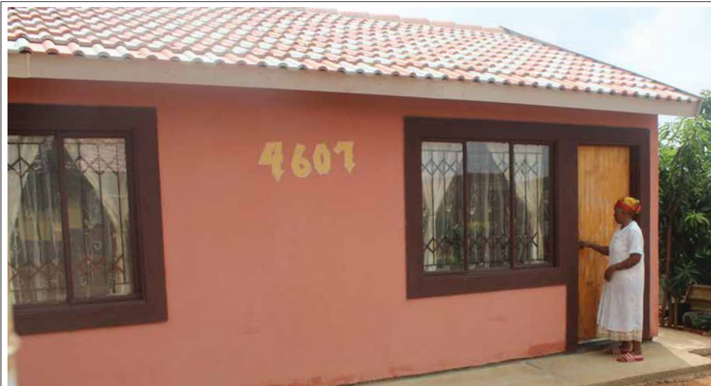
Some 500 residents from Hammanskraal have benefited from a housing project of the Gauteng Department of Human Settlements.
