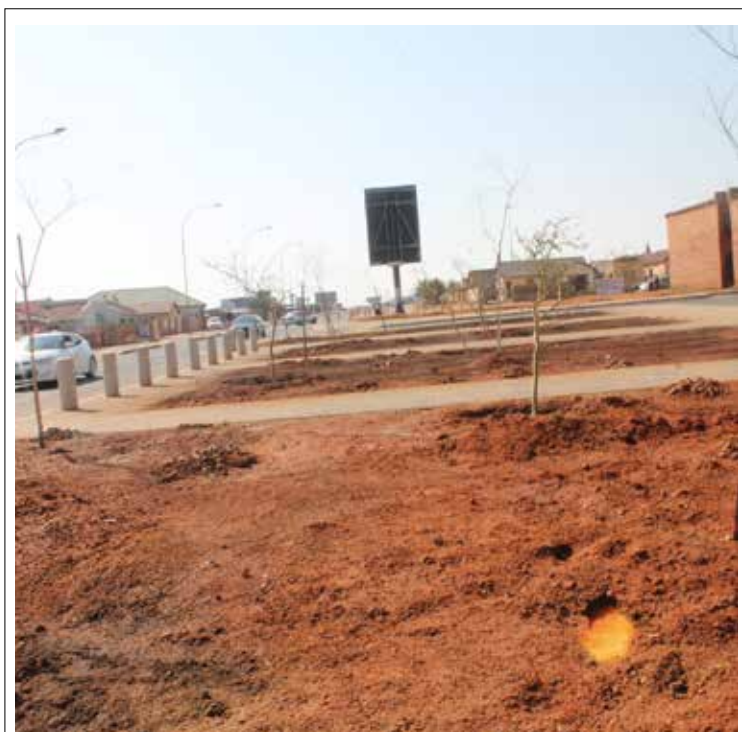
■ Upgrading the sidewalks in Mohlakeng.
