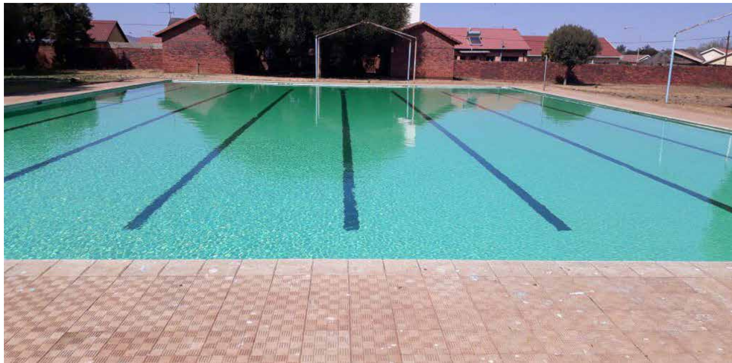
■ City of Joburg swimming pools are being refurbished to keep residents cool and entertained.
