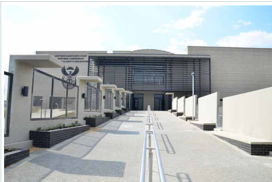
■ The new Booyens Magistrate's Court comprises of ten court rooms which makes access to justice easier.
