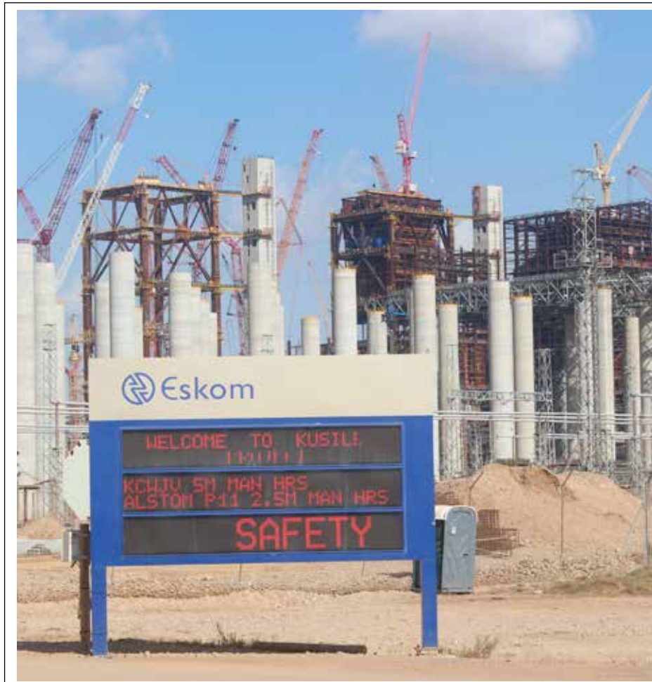
Kusile Power Station, currently under construction Mpumalanga, is expected to open in 2019 and help ease the country's electricity demands.
