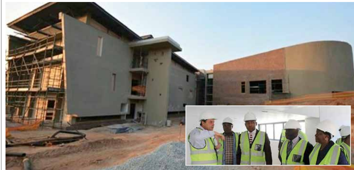
Deputy Minister of Higher Education and Training Mduduzi Manana recently visited the University of Mpumalanga in Mbombela to assess the construction of the new buildings.
