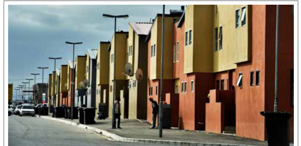
The N2 Gateway Integrated Human Settlements Development project has delivered more than 14 000 houses.
